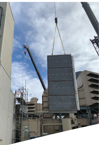
Replacement of silencer baffles.
