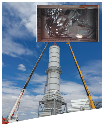
Emergency removal of failed baffles.
