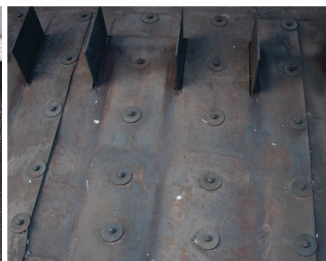
1) Damage to the silencer floor discovered during outage.
